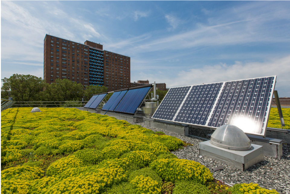
NYC DDC – Green Roofs, Creating a More Sustainable New York City
